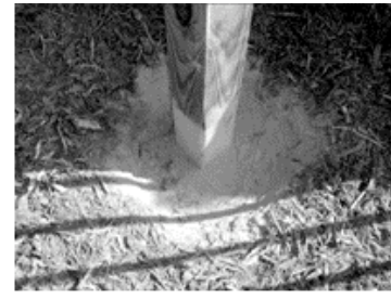
Install Pole using concrete
