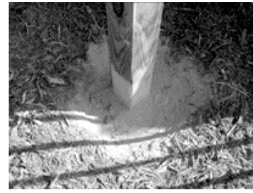
Install Pole using concrete
