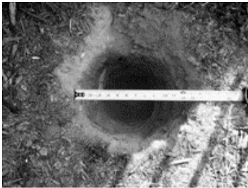
Dig Hole with 8" Diameter
